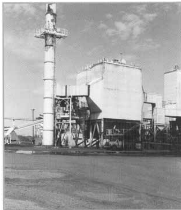
This 22-MW stand-alone, biomass fired power plant at Pacific Oroville Power Inc., Oroville, California, burns about 450 to 500 bone dry tons of wood chips and other fuels per day at full capacity.
