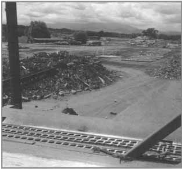
Overlook from debarker to yard at the small log mill of Sierra Pacific Industries, Anderson, California. The cogeneration plant uses woodwaste from lumber and pole manufacturing to produce electricity for the mill and office and heat for the dry kiln.
